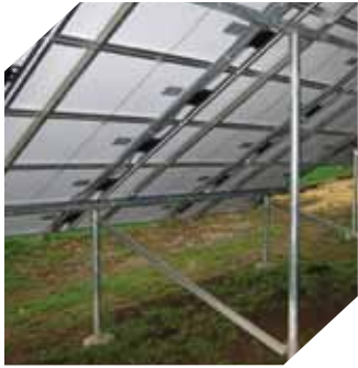
Underside of large ground mount
